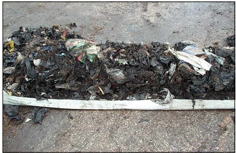
Airlift - Plastic removed and contained in discharge sock
