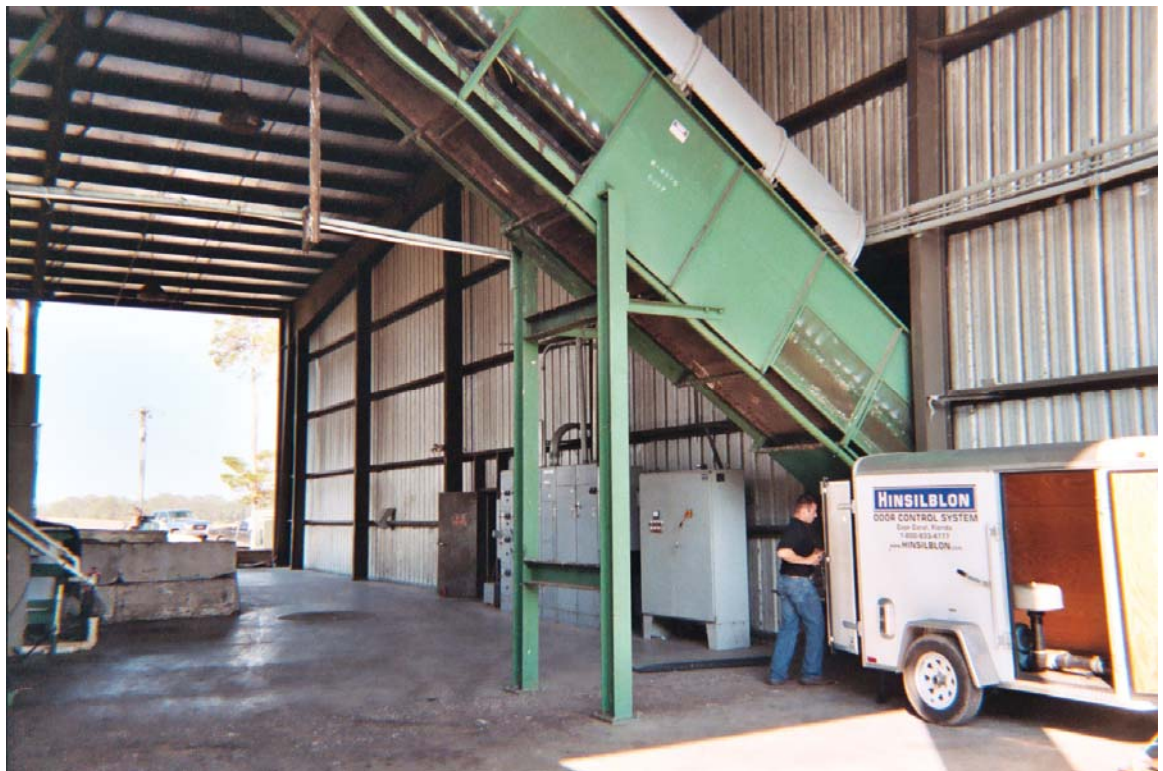
HDLA300 System During Installation
