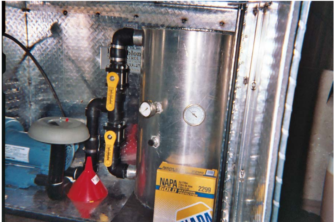
HDLA100 System during installation
