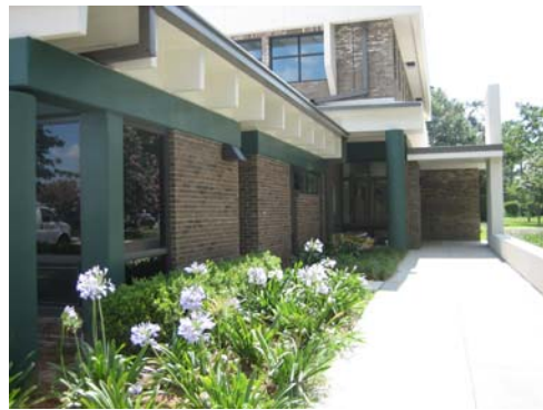
Front of Building – left side view
