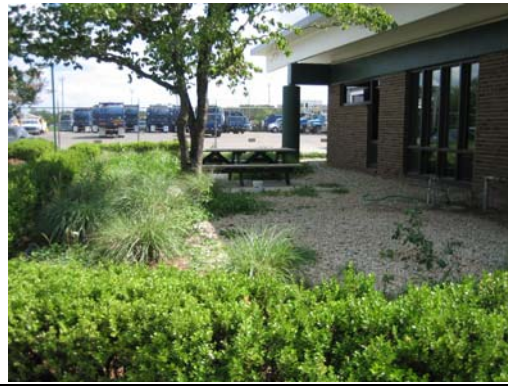
Side of Building – corner left side view
