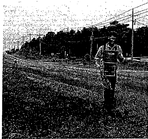
Mulch is applied to roadside after seeding (above), while grass seed is hand applied to strip supplied with compost (right). Seeding with compost and hydroseed fiber (below) has been effective for sediment control.
