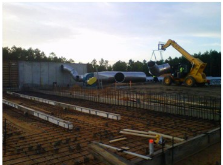
VISTA Under Construction
