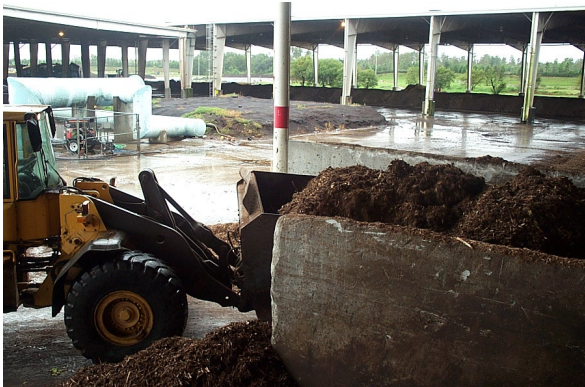
Mixing in Concrete Bunker
