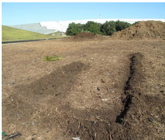
Berm is created to contain material in designated area.
