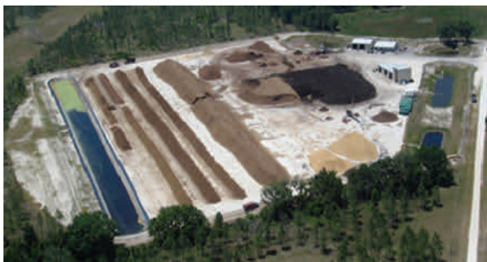
C&C Peat Composting Facility
