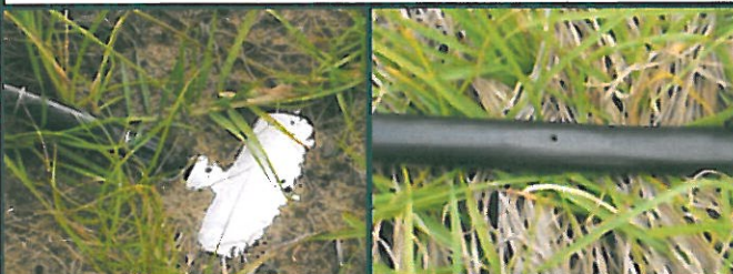
The Newly Installed Netafim USA Irrigation System
