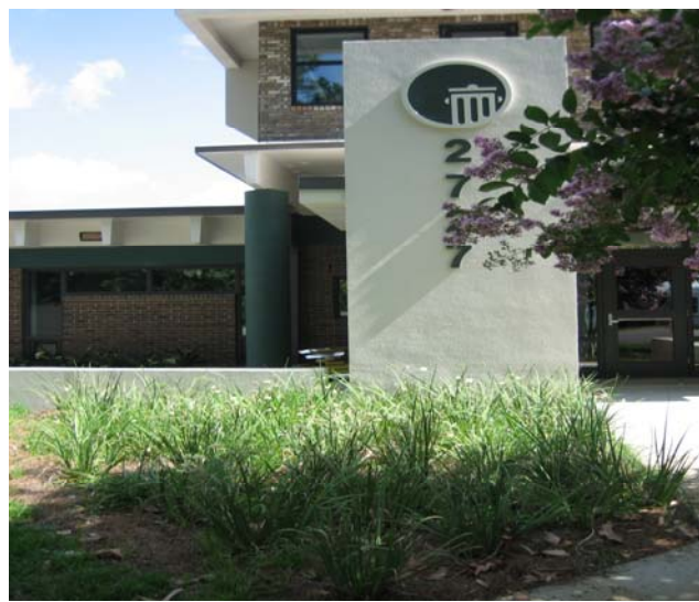
Renovated Building Entrance
