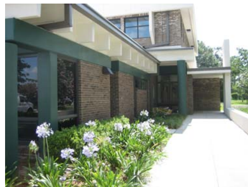
Front of Building – left side view
